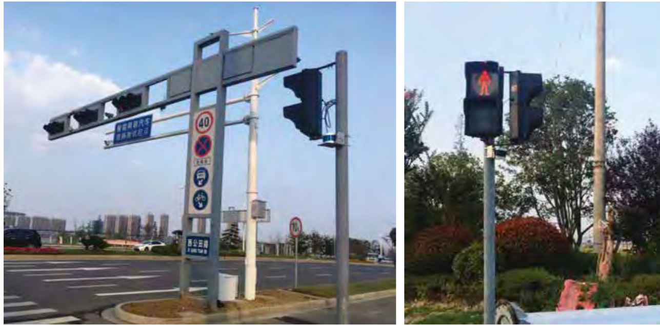
Figure 3-16: 5G vehicle-road synergy demonstration zone in Suzhou High-Speed Rail New Town
