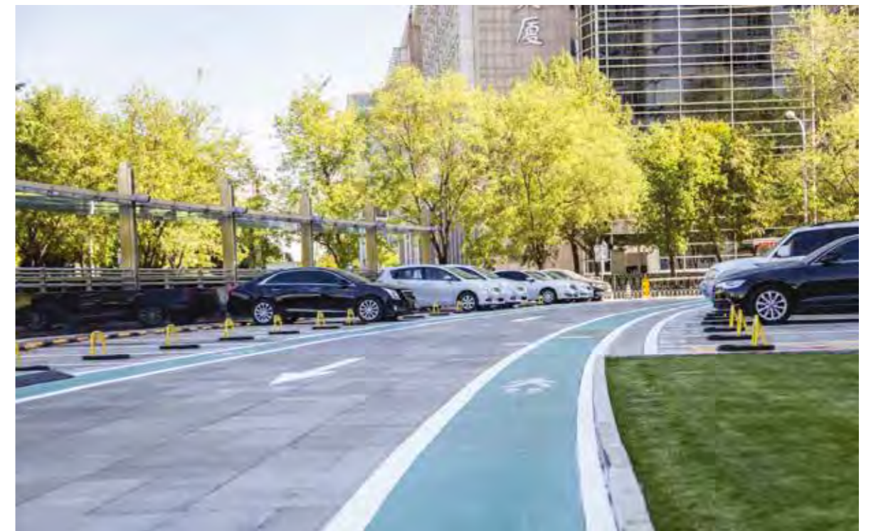
Figure 3-15: 5G networked automatic parking in Shanghai
