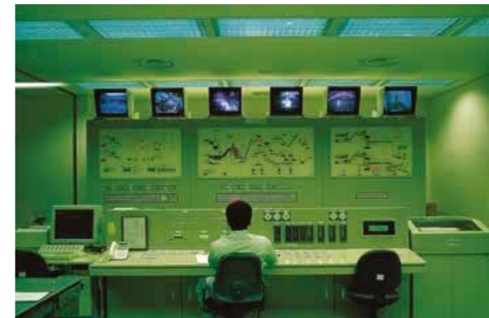
Figure 2-14: 5G-based underground device data collection
